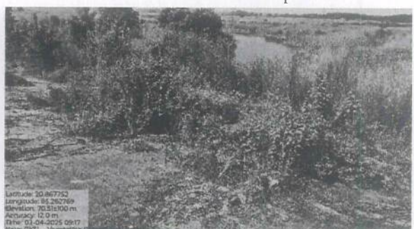
Vegetation Growth on U/S Slope and Pooling of Rainwater
