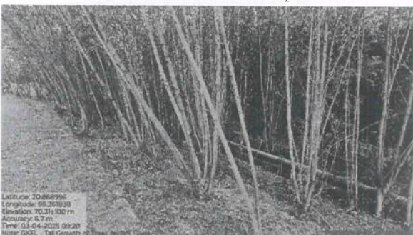
Tree Growth on D/S slope at Certain Sections
