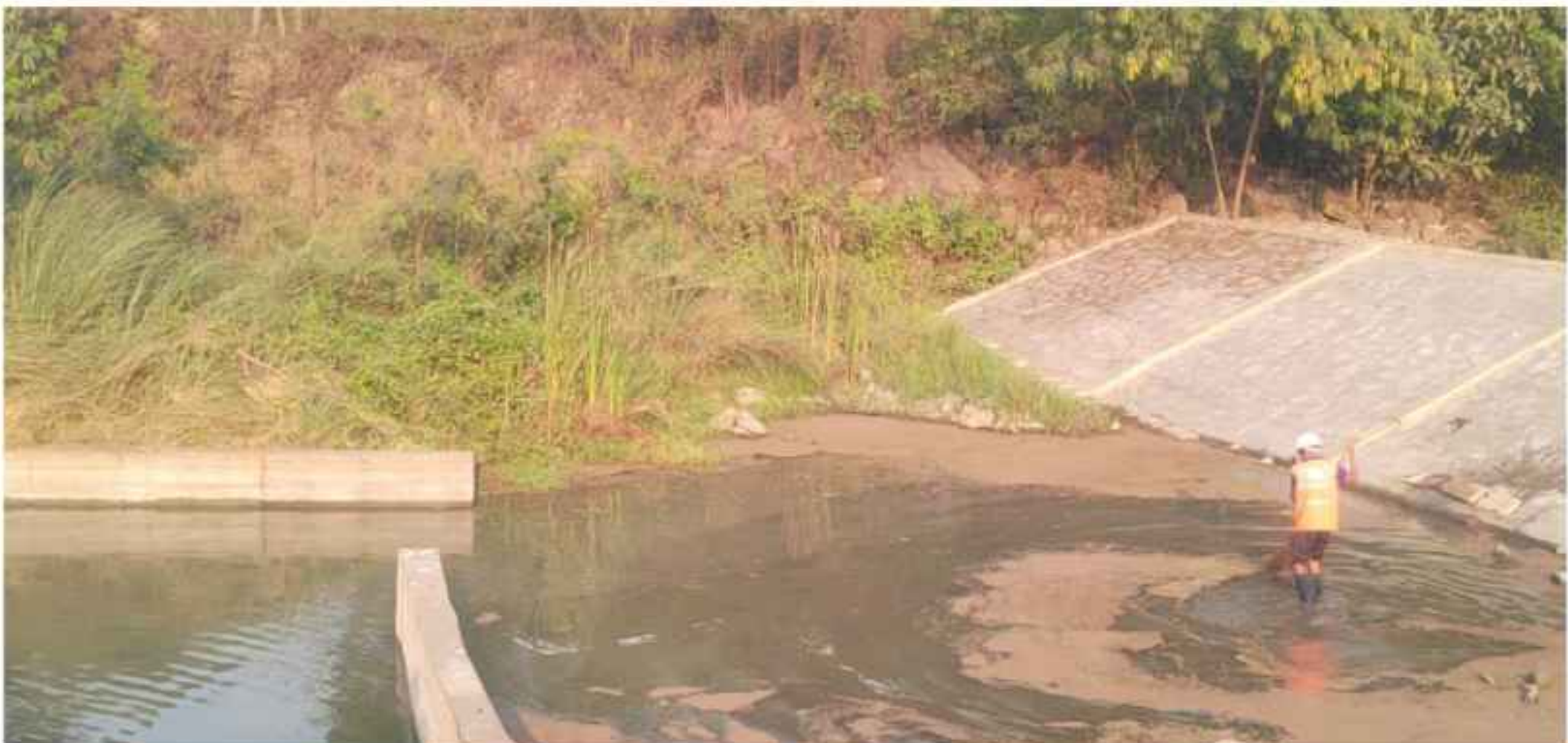
PHOTOGRAPH-6, ADDITIONAL SPILLOVER POND
