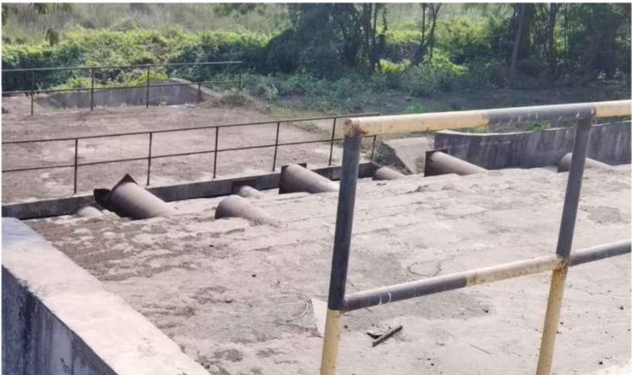
PHOTOGRAPH-4, SPILLWAY DOWNSTREAM VIEW
