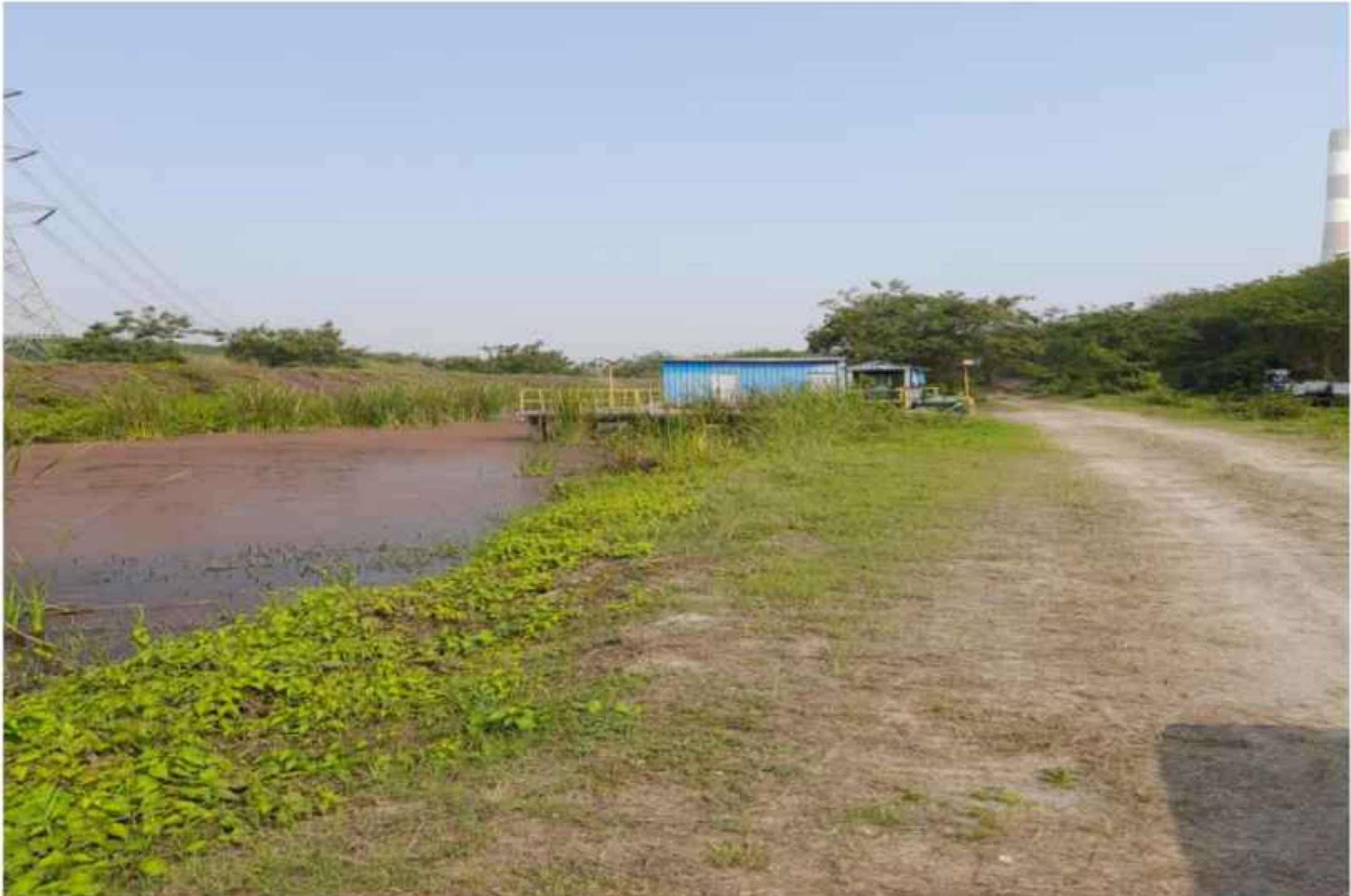
PHOTOGRAPH-5, RECOVERY PUMPHOUSE
