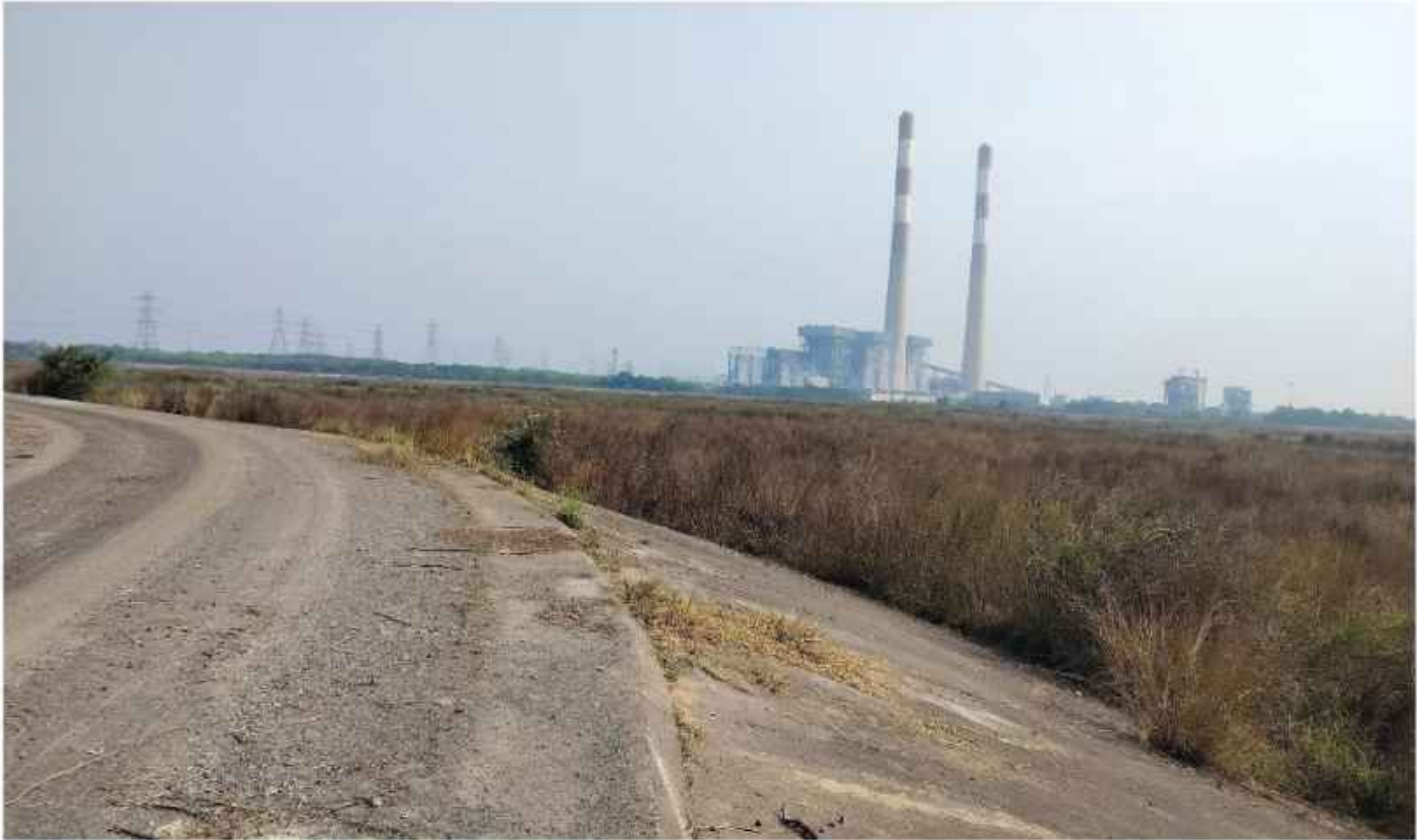
PHOTOGRAPH-3, ROAD OVER DYKE & UPSTREAM SLOPE LINING
