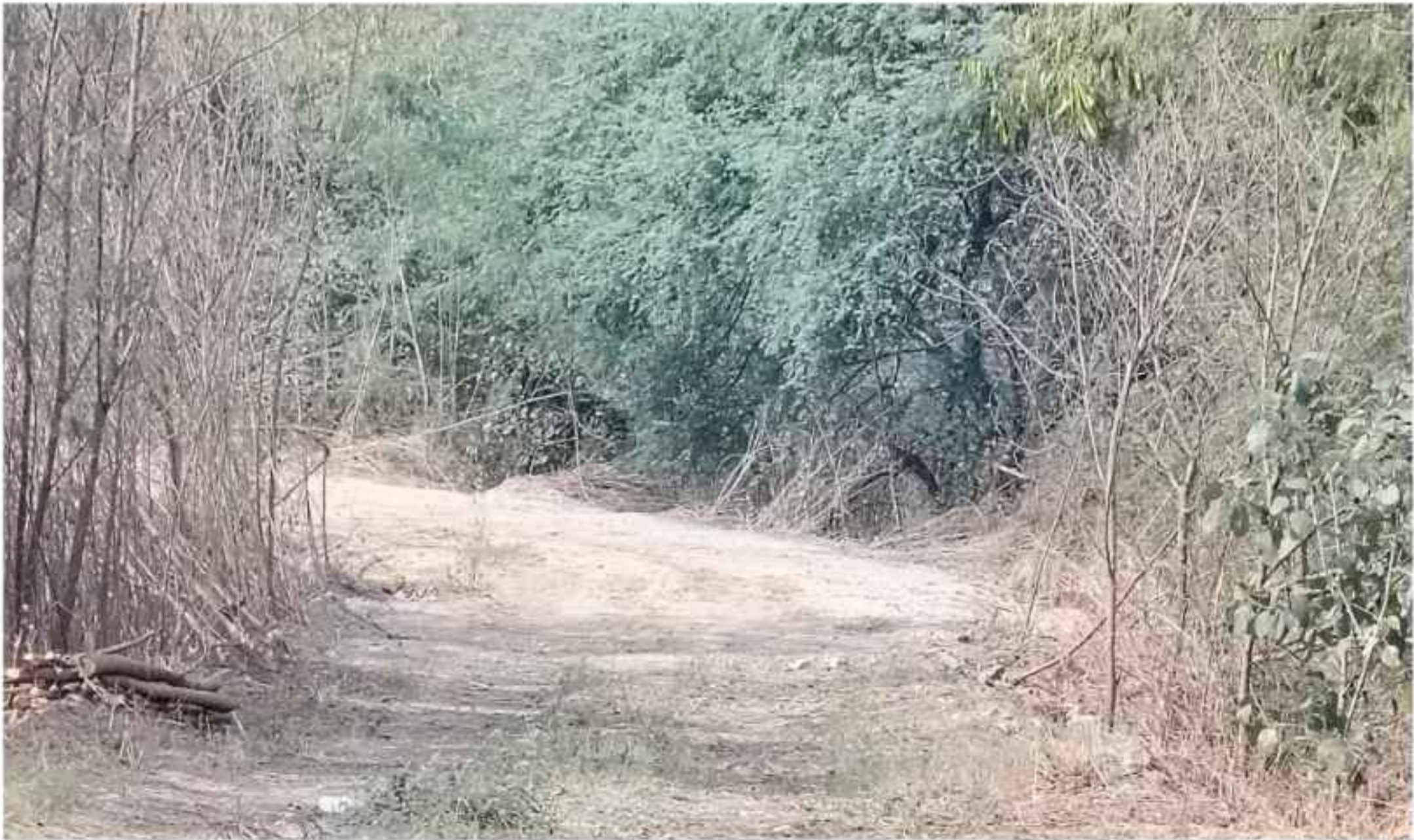
PHOTOGRAPH-2, ROAD OVER DYKE TOP WITH GREENBELT OUTSIDE
